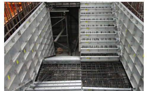
12 Setting staircase panels
