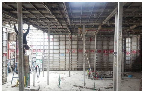
10 Setting slab panel
