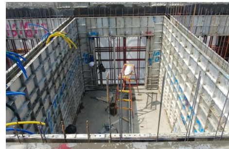
07 Setting wall panels
