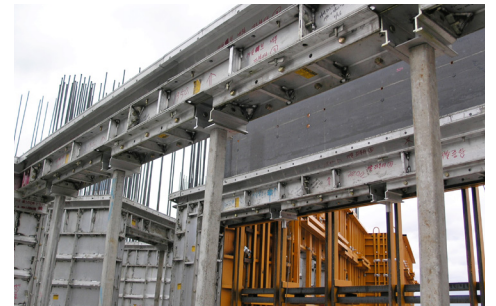
08 Setting S/L and beam panels
