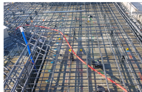
15 Rebar works for slab
