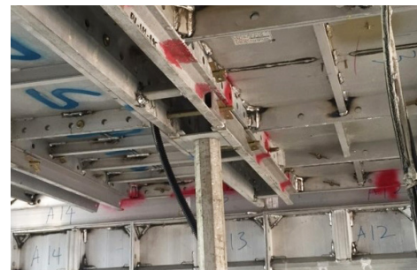
11 Setting slab panels
