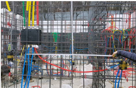
05 Checking rebar works
