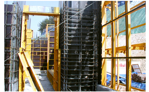
04 Rebar works for wall
