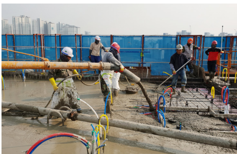
17 Concrete Casting
