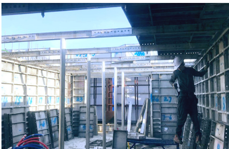
09 Setting slab beams
