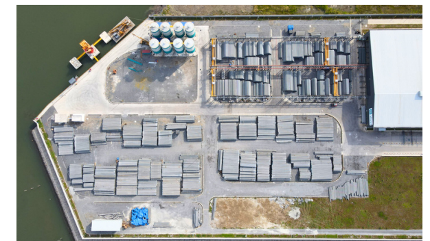
Stock yard / Bãi cọc
