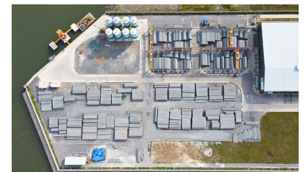
Stock yard / Bãi cọc
