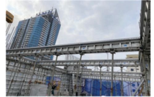
08 Setting S/L and beam panels
