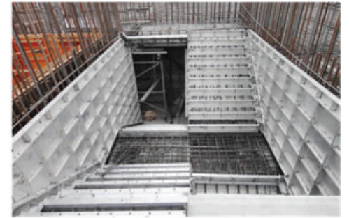
12 Setting staircase panels
