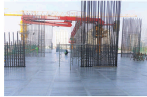
11 Setting slab panels
