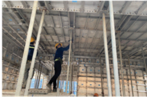
10 Setting slab panel
