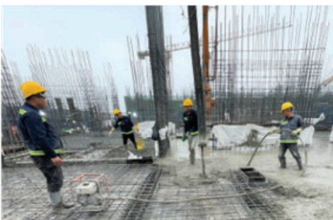
17 Concrete Casting
